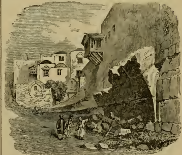
No. 1. — Remains of Arch of Bridge. (S. W. angle of Haram.)
