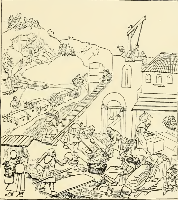
BUILDING OF THE CISTERCIAN MONASTERY, SCHÖNAU, NEAR HEIDELBERG.
